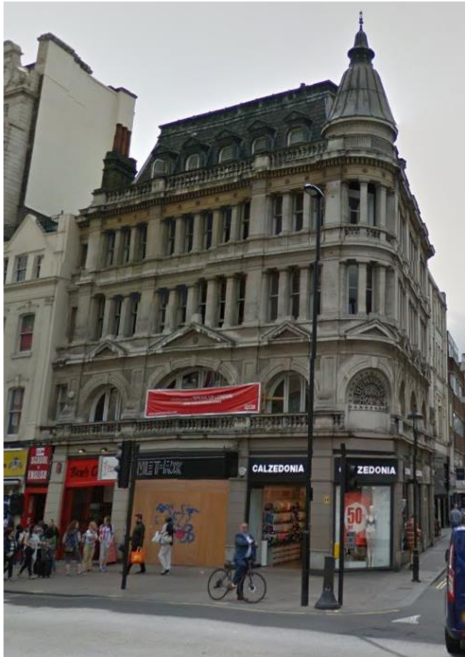
Site 1: Berwick House, 139-143 Oxford Street, London, W1D 2JA
