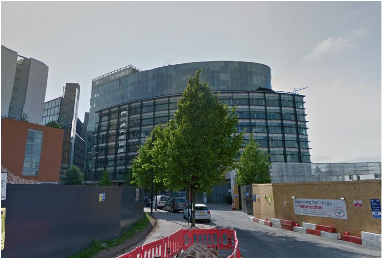
North elevation from North Wharf Road.
